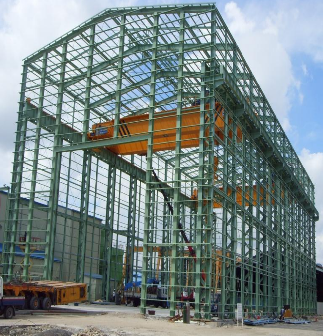
HEAVY WALL SHOP 철골공사
