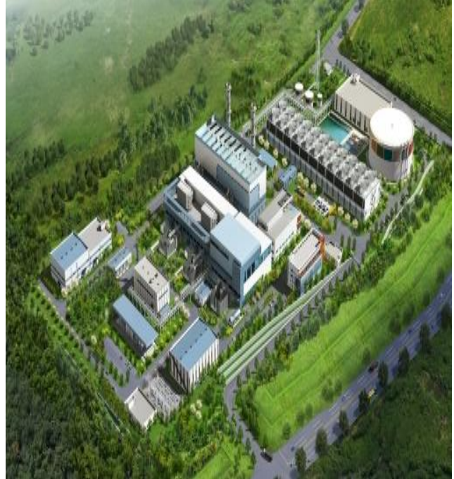
울산 GPS CCPP Project
