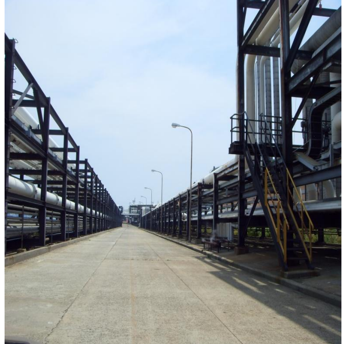
SK Gas Tank Terminal 철골공사-" I " AREA
